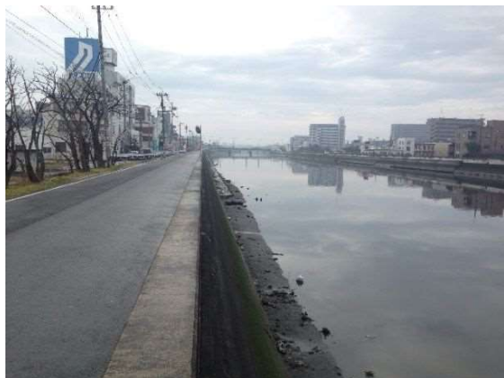
詰田川耐震化前
