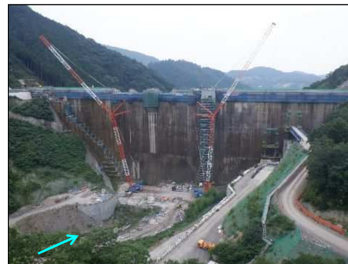
Co打設完了時(R2.7.31)
